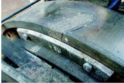
Kiln Tyre Crack Repair
