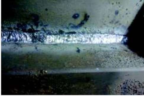
Arc Furnace Shell Crack Repair
